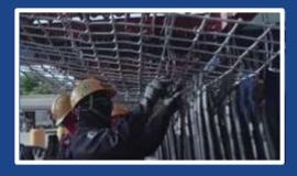
All fabricated steel that enters an SCG galvanizing plant for processing is thoroughly inspec- ted to ensure drainage and venting requirements are met.
