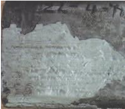
Figure 1: De-lamination
