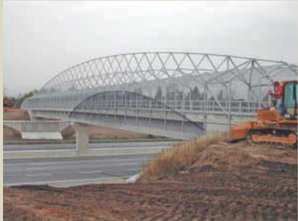
Morningside Pedestrian Bridge Location: Cambridge, ON Date Galvanized: 2008 Project Maintenance: 95 years
